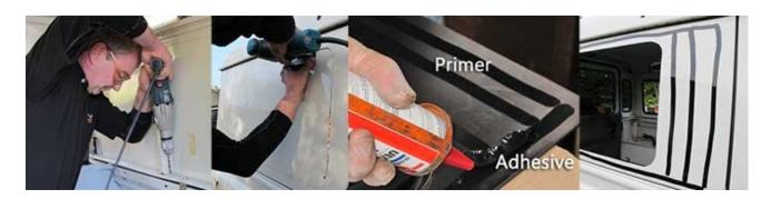
Once you are confident you can cut out the aperture accurately, drill a hole for the blade near the marked line, within the marked area in the chosen place you want to start cutting.
